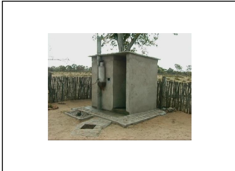
Fig. 13. Makoni District, (2001) MoH standard Blair latrine model with built in hand washing facility
