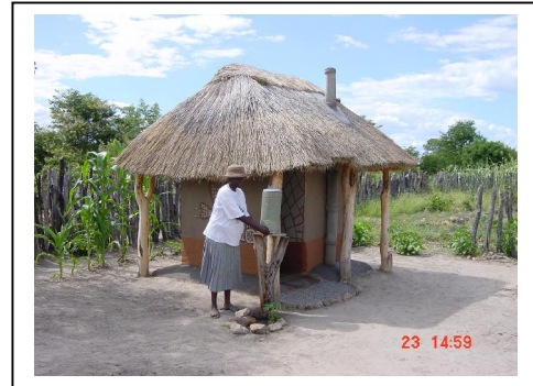
Tsholotsho District, (2001) Mud and pole Ventilated Latrine with free standing hand washing facility
