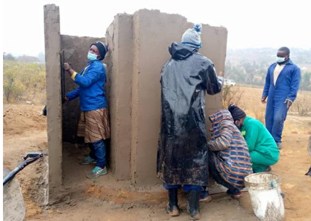
Photo: Annastancia Gwata ( entrance ) taking part in the latrine builders training in Ward 13 of Mutasa District. CARE International, July 2020.
