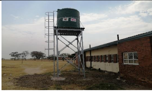
Tank and stand installed at Gwabalanda ECD
