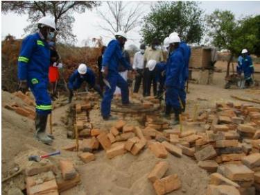
Fig 2 latrine builder training - ward 12 - Gutu
