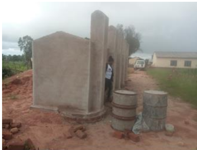
Fig 3 School latrine construction at Chokera School in ward 12 and Mugodhi in ward 36
