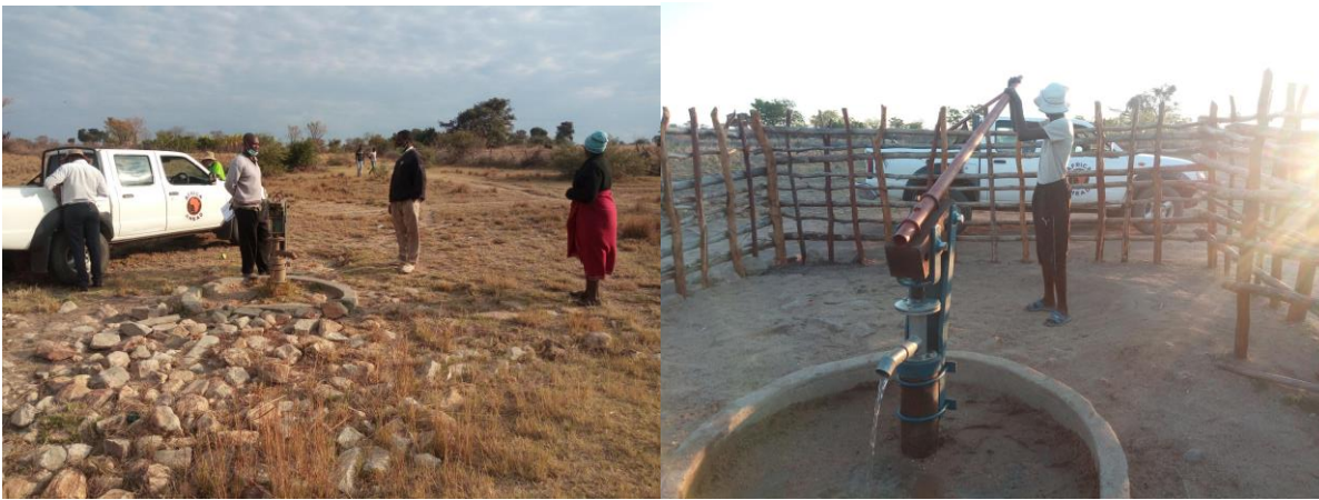
Fig 5 Borehole rehabilitation - Before and after of Gijima water point in ward 12 - Gutu
