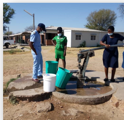
Above: Water points at health facilities repaired including new storage tanks and repair of handpumps.
